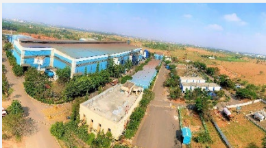
Utilizing wind power and solar power
