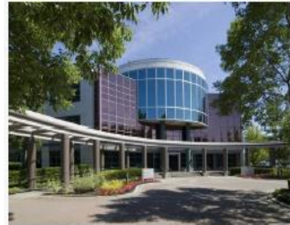
Photo : Wenco Office Building (Richmond, BC, Canada)
