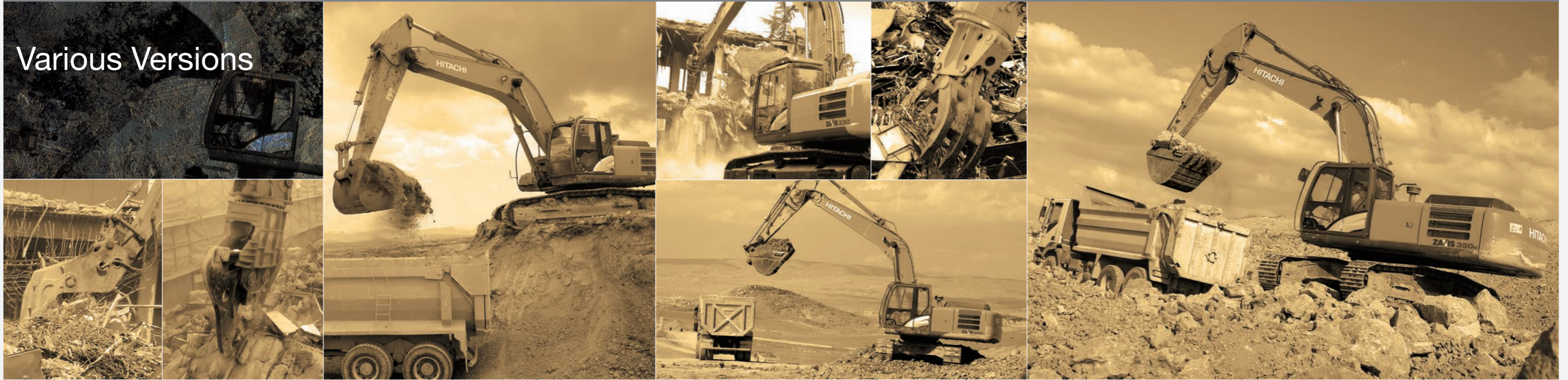
The photos above show machine images at work, which include machines other than ZAXIS 330 series.
